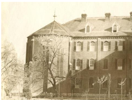
Motherhouse, Original north wing with chapel, constructed in 1874
