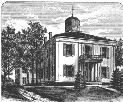
Schiller Mansion showing small dorm to rear—the first home of St. Elizabeth Academy
